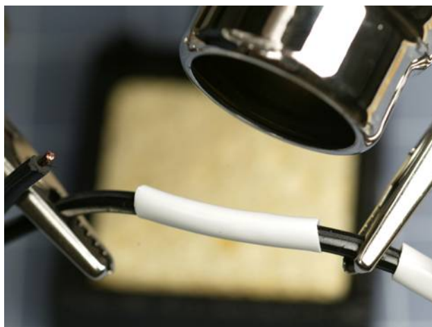
Figure 3-57 Step 9 of 12, to shorten a power cord.
